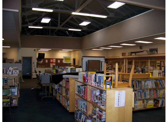
Main building (265A), media center (former boys gymnasium) with exposed truss system, looking west.
