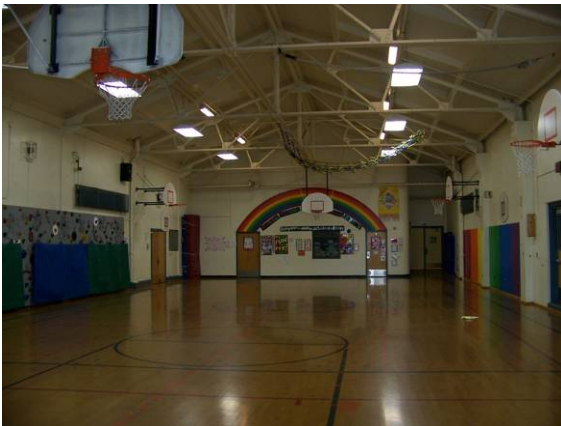
Main building (265A), gymnasium, looking west.
