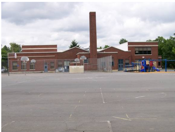
Main building (265A), east (rear) elevation, looking west.
