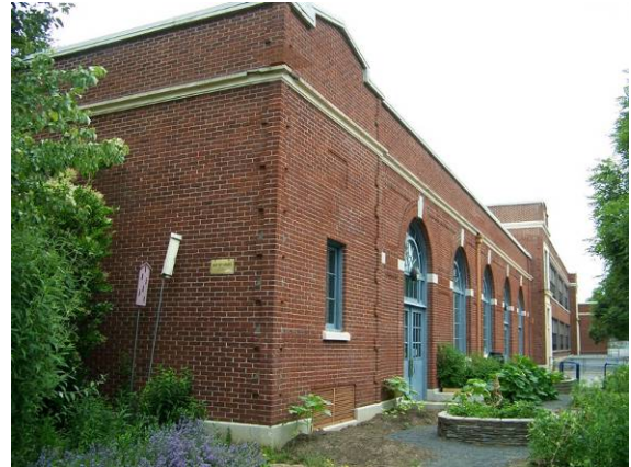
Main building (265A), south (side) elevation, looking eastward.
