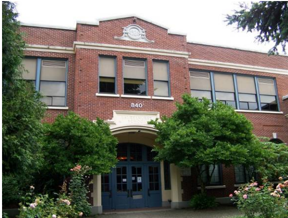
Main building (265A), west (front) elevation, looking eastward.
