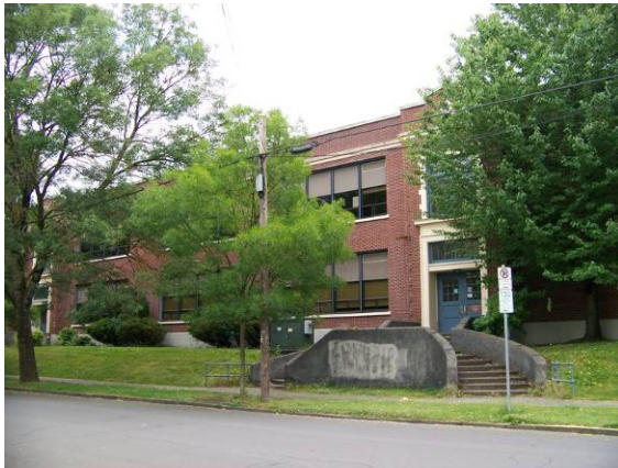
Main building (265A), north (side) elevation, looking southeast.
